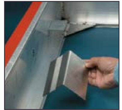
Permanently attach brackets and stiffeners.
